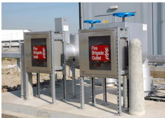
West Box Portal Breaching Point
